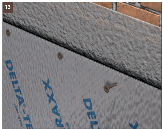
(Fig. 13) If the grade line is known, the sheet may be fastened immediately using DELTA ® -MS DÜBEL.
