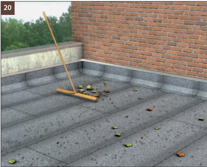
(Fig. 20) Clean waterproofed surfaces thoroughly so that the waterproof coating cannot be damaged after the drainage sheets have been laid out. If the roof is to be planted later on, the waterproof coating must be root-resistant or shielded against root penetration with a protective sheet.
