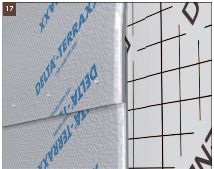
(Fig. 17) Join the two parts with at least four DELTA® adhesive pins.
