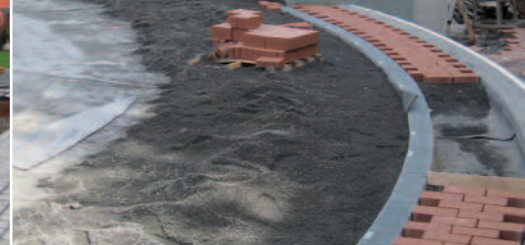
Sub-base being applied on top of DELTA-TERRAXX.
