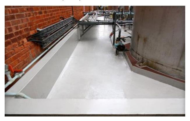
Epoxy Bund Paint is a tough, flexible, chemical resistant and waterproof epoxy resin coating for concrete and metal bund tanks. Suitable for internal and external surfaces. Chemical storage bund areas, balconies, flat roofs, metal stairways, gutters and all other areas requiring waterproofing and high chemical spillage resistance.
