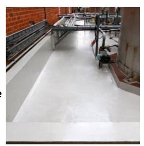
**BUND PAINT** is a twin pack epoxy resin coating. When fully cured, the material provides a flexible, abrasion, chemical resistant and waterproof coating of outstanding durability for both interior and exterior applications.
