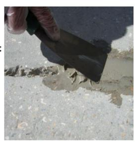
**Epoxy Filler** is a twin pack epoxy resin for permanent repairs to cracks and holes found in concrete, stone, tiles and brickwork.
