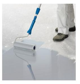
**EPOXY SEALER** is a two-part, solvent free, epoxy resin for sealing and impregnating concrete floors that demand outstanding performance. A tough, durable, chemical resistant surface that are easy to clean. The glazed finish is capable of withstanding heavy fork trucks and intense pedestrian trafficking.
