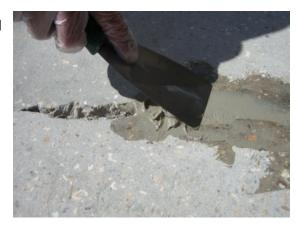
**DESCRIPTION:** Epoxy Filler is a twin pack epoxy resin for permanent repairs to cracks and holes found in concrete, stone, tiles and brickwork.
