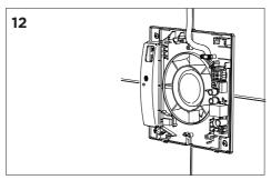
Route the cable and secure within the fan.
