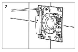
Ensure the fan is level and then mark the 4 mounting holes.
