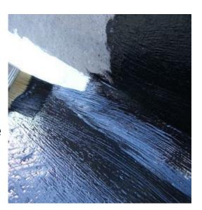
**DAMP PROOF MEMBRANE** is a flexibilised epoxy resin coating. When fully cured will provide a chemically resistant, water and vapour proof coating suitable for both interior and exterior applications.
