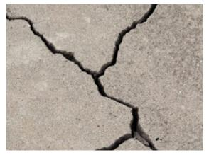
**DESCRIPTION:** Epoxy Crack Repair T is a high viscosity, thixotropic, two part, solvent free, epoxy resin paste for sealing wide cracks found in concrete, brick and stone and for wall tie placement. This product exhibits superb early strength development and adhesive power.
