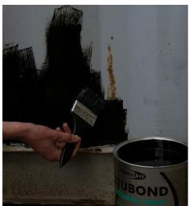
soft and less resistant to degradation by the environment, and will ultimately flow. It is important that the first coat is completely dry before application of the second coat.
