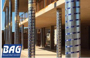
A single use, water resistant cardboard former providing a smooth fair faced finish on circular concrete columns. Column formers are manufactured in the UK, to your specific length. Interdrated tear off strip allowing easy removal. They can also be placed around the completed columns for protection.
