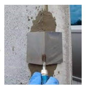
**EPOXY MORTAR LIGHTWEIGHT** is an incredibly tough epoxy resin lightweight mortar ideal for repairing eroded or damaged concrete or stone window cills, columns, beams, lintels and overhead concrete ceilings. It has outstandingly high strength and chemical resistance. Similar product to our standard Epoxy Mortar with the advantages gained by being lightweight.
