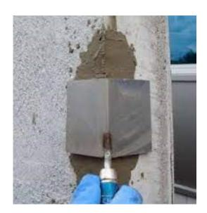
EPOXY TACK PRIMER VG is a two part, solvent free, epoxy resin primer and adhesive designed primarily as a primer to be applied vertically prior to applying our Epoxy Mortar. The adhesive strength and performances are exceptionally high and therefore make it an excellent product in its own right for filling cracks found in concrete walls.
